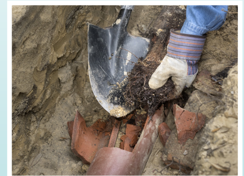
Plumber making repairs on private lateral
