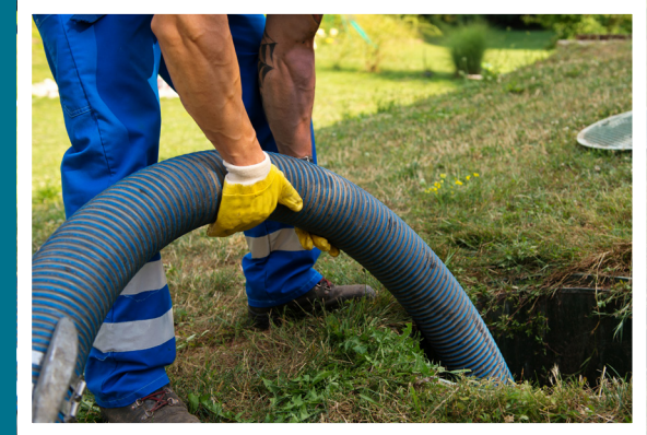
Tank being professionally pumped.
