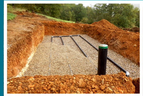
Drain field being installed.
