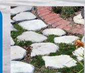
runoff to infiltrate through the soil and prevents most pollutants from eaching the storm drain system.
